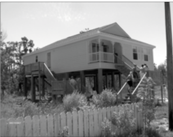
A 1400 sq. ft. affordable home just built in Mississippi. It is elevated to meet new building requirements.
